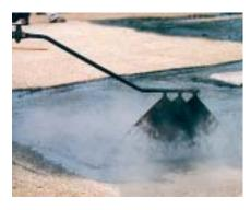
Versatile handspray attachment is standard equipment, allows greater efficiency on all maintenance jobs. For finishing intersections, patching, and surfacing in limited areas. Includes hand spray gun with triple lap 3 nozzle spray and 25' of asphalt grade hose.
